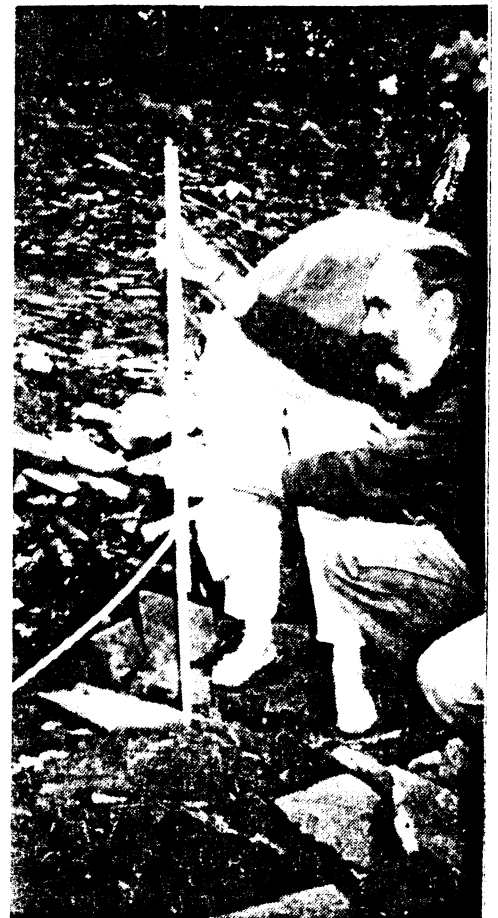
Course fare: laying out swales with a water level.
