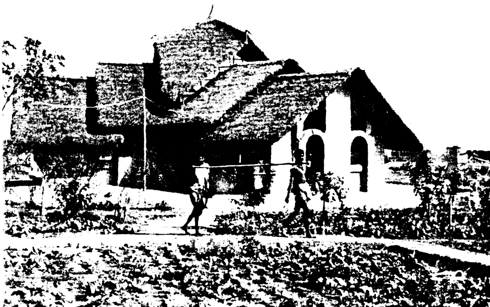
Built of local materials with local skills. Thatchers guaranteed the roof for 11 years. The bricks are unfired.
