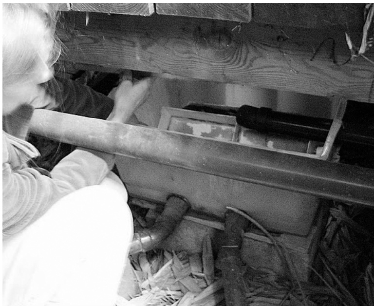
The urine and flushwater dosing chamber. This assures the “yellow water” from the toilet has time to get absorbed into the grey-and-yellow water system before another pulse drains into it. The chamber also assures there is some velocity for every dose.
