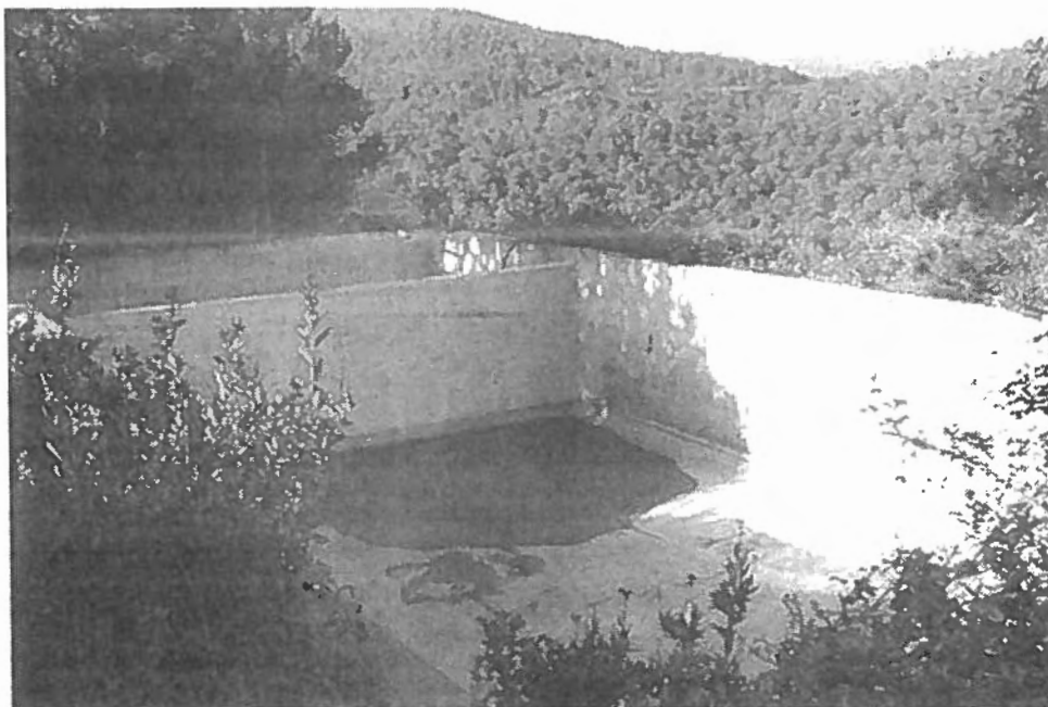
One of half a dozen ferrocement water tanks on the property hold winter rainwater through the long, dry summer. The region is in the third year of a harsh drought.
