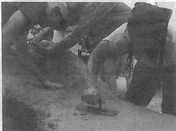
Troweling a plaster coat onto a cob bench
