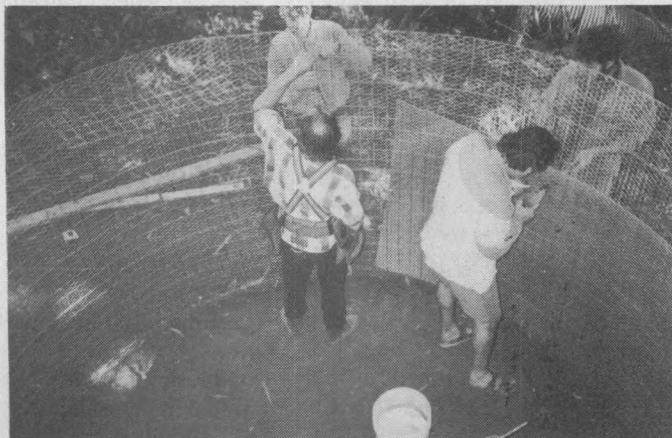
Tying the reinforcing mesh and attaching masonite sheets.
