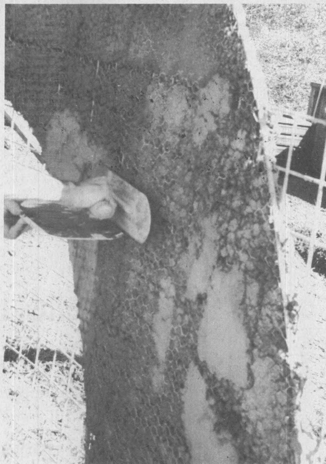
Applying plaster to the mesh form.
