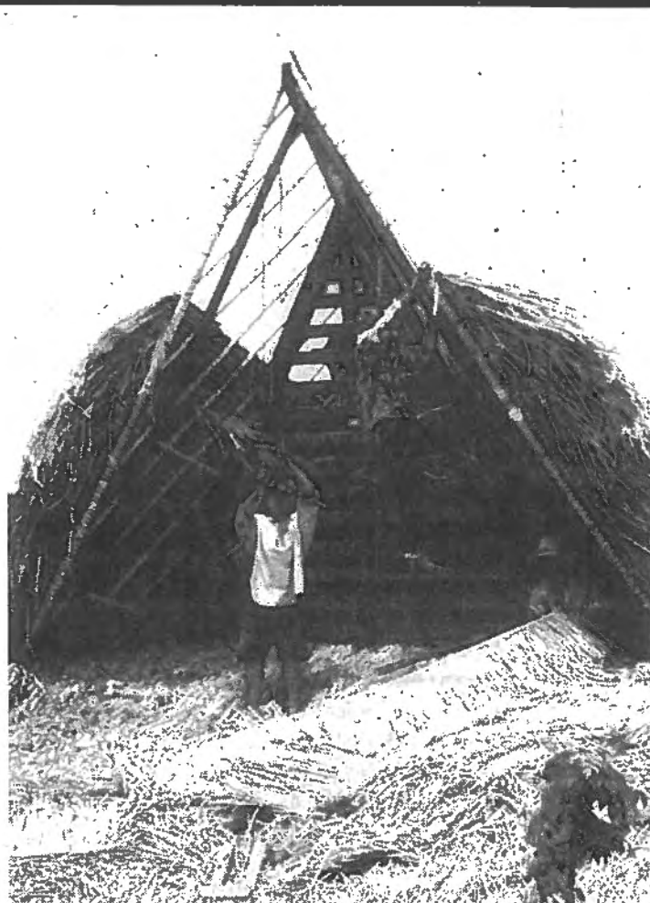
Steep sides and thatch shed rainwater off this house in Java.
