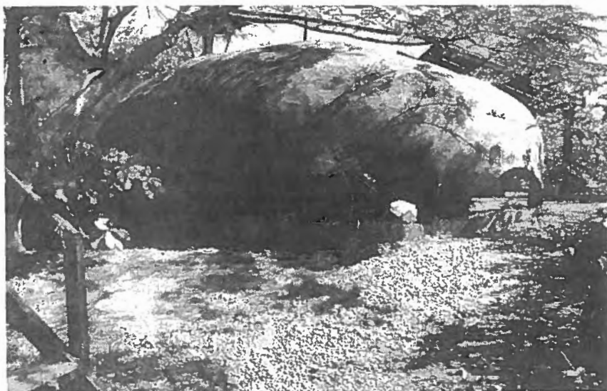
The elegant curvature of natural forms infuses the design of this ferrocement shower block at IPEC, central Brazil.
