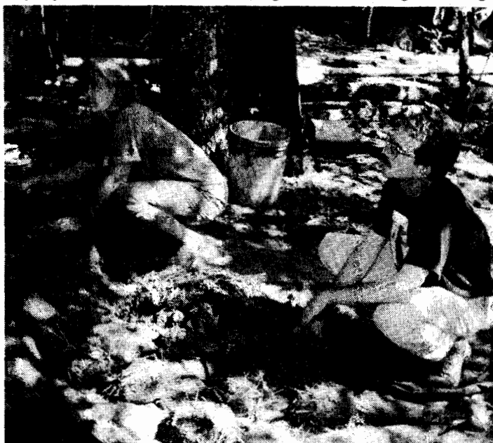
Cob is formed from soil and sand to which chopped straw is added. The loaves or cobs, are worked into the wall.
