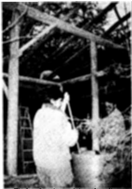
Timber framing; mixing clay slip
