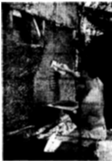
Applying earth plaster to a clay-straw wall which has been slip-formed
