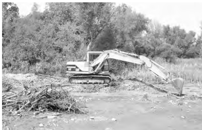
A track-hoe was the right tool for the job, requiring less than six hours to build the chinampa beds.
