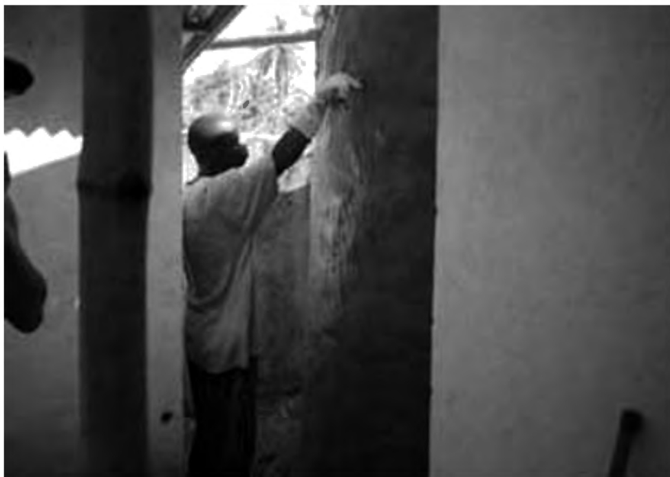
Putting on the render coat, Lassana Kamara was our quality control man for this process of the tank construction.
