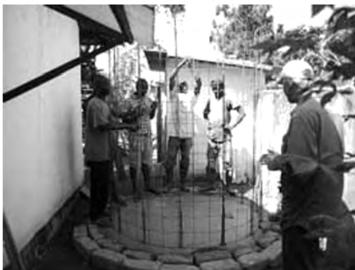
Framing the inner structure for the ferrocement cistern.
