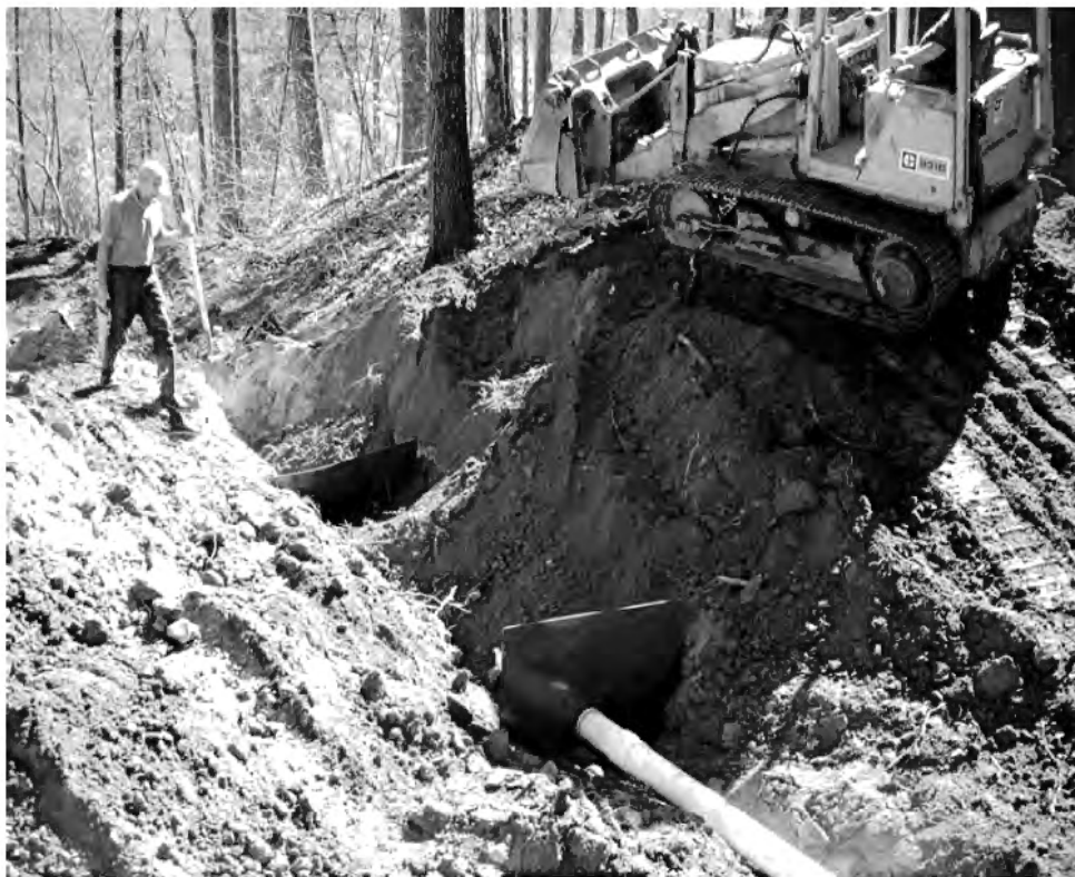
The author examines the pond's drainage line during installation. Rectangular baffles along the pipe will prevent laminar flow of water and potential failure of the dam.
