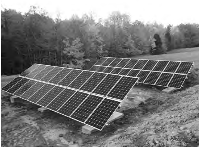
Ground-mounted solar array facing southwest to take advantage of the utility's time-of-use crediting.
