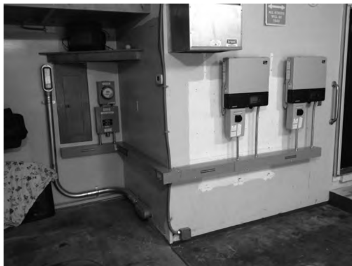
A typical balance of systems (BOS) set-up including two inverters, a subpanel, and a production meter, tied into the existing electrical service.
