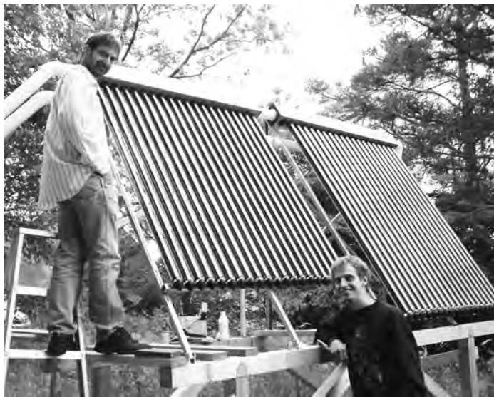
Husband Chris (L) and brother Mark (R) finish installing evacuated tube collectors. We tested two different models of collectors. Both perform well, and will be installed in new Passivhaus.
