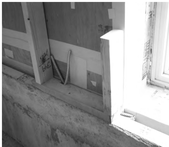
In my Passive House, the air-barrier layer in all wood-framed walls is plywood with all seams, corners, and knots and fasteners taped as shown here. All electrical lines will run in a 2x4 wall inside of the air barrier (mocked up in photo) with additional batt insulation.
